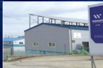
TANK LINING FACTORY (Eum-Sung)
